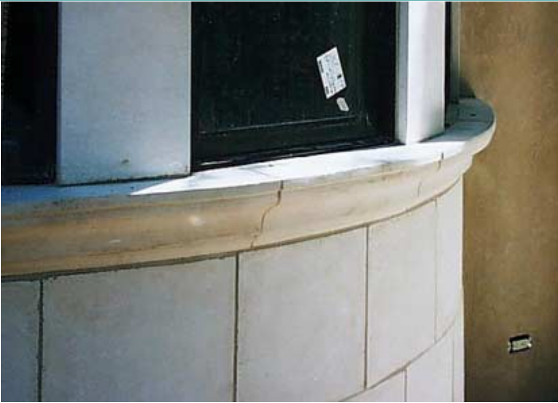
Curved Sills and Cladding
