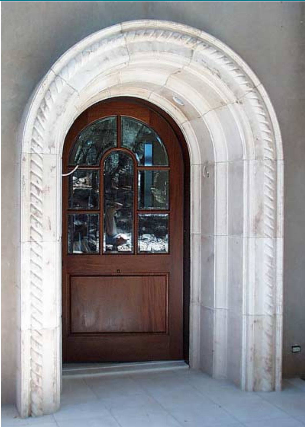
“Architrave”, “Porte Cochere” made out of heavy moldings This front door treatment is impressive. Next page for the specifications
