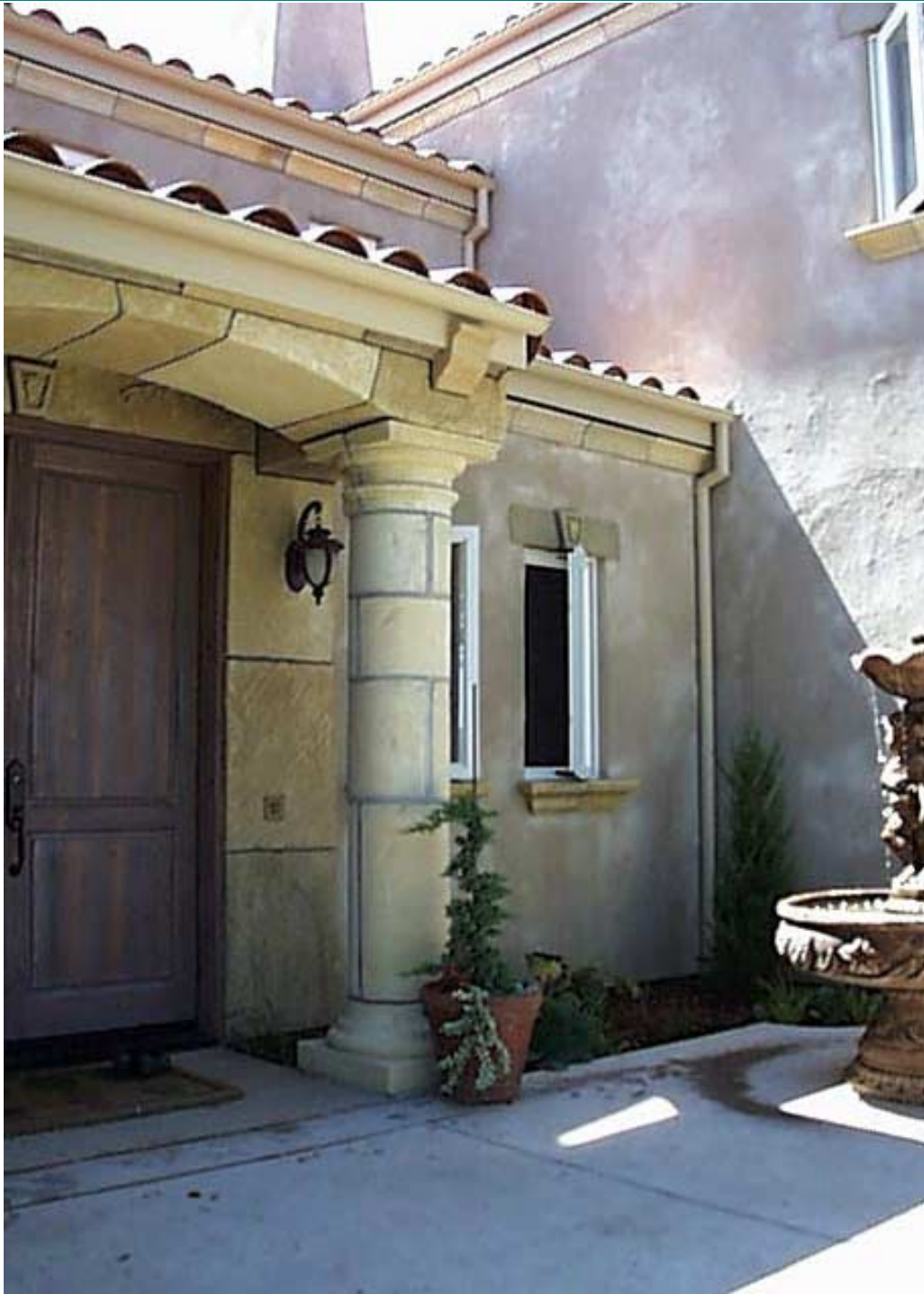
Eave moldings, Window Sills...
