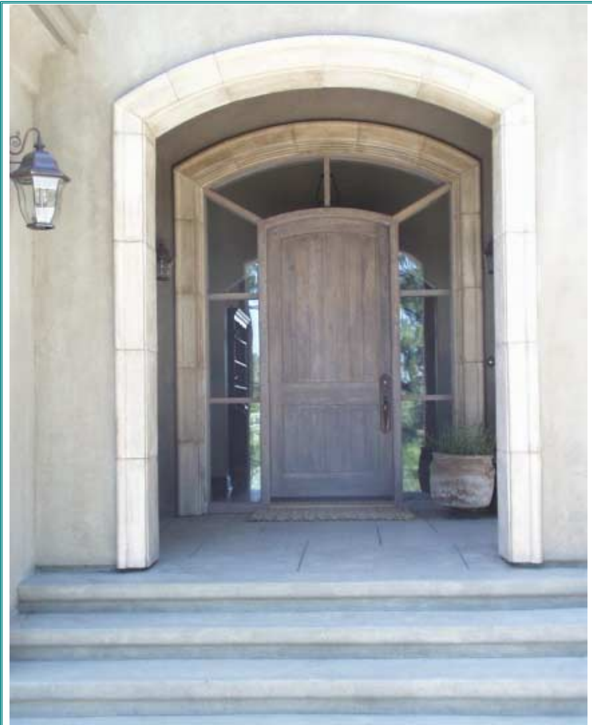
Front arch made with stepped cove and the window Bull molding
