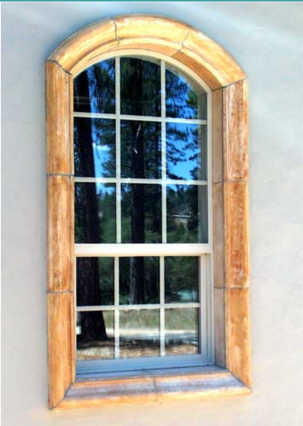
Notice the curved cladding on the radius assembly
