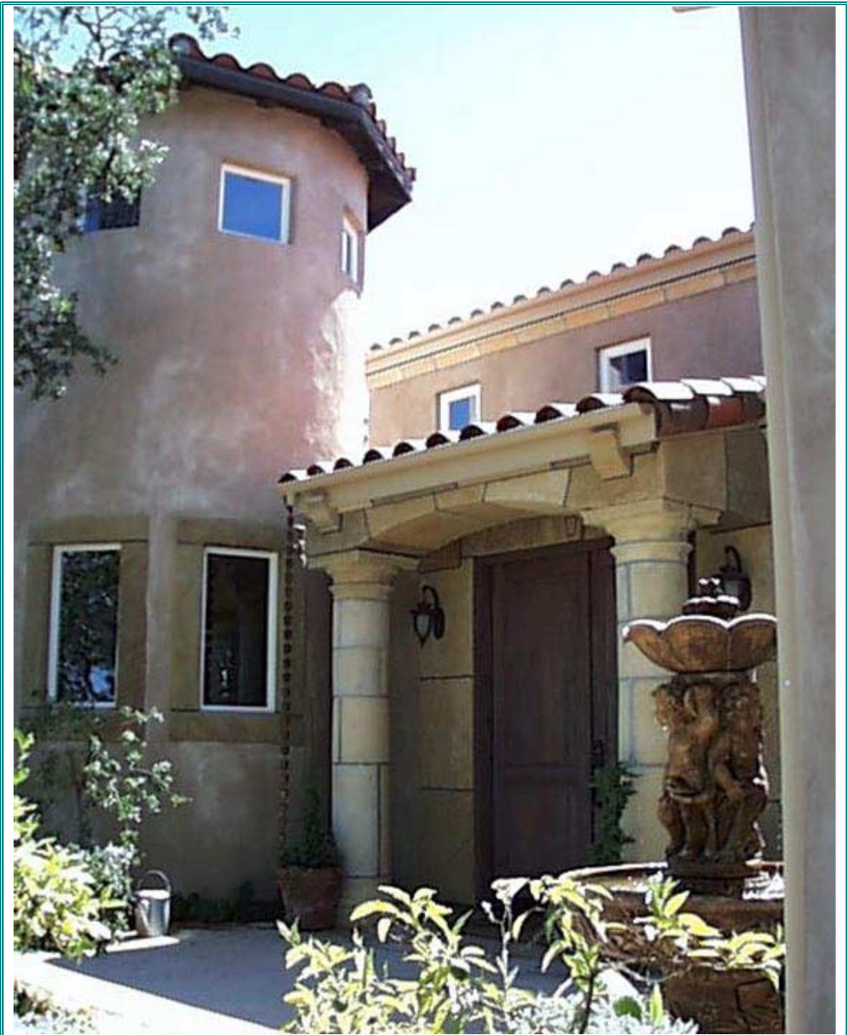
Front Porch Eave Moldings
