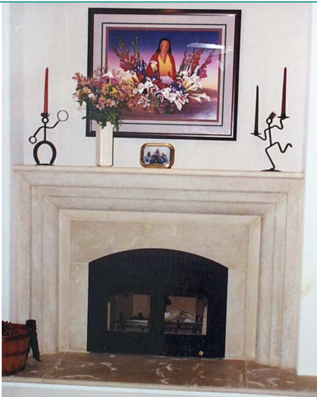
“Logsdon” Bolection This Bolection is 70” long. It has to be mitered and cut to specs
